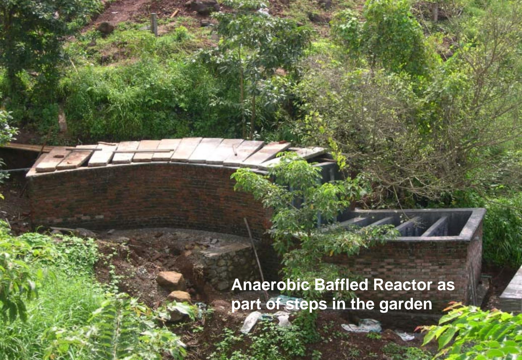
**Anaerobic Baffled Reactor as part of steps in the garden**
