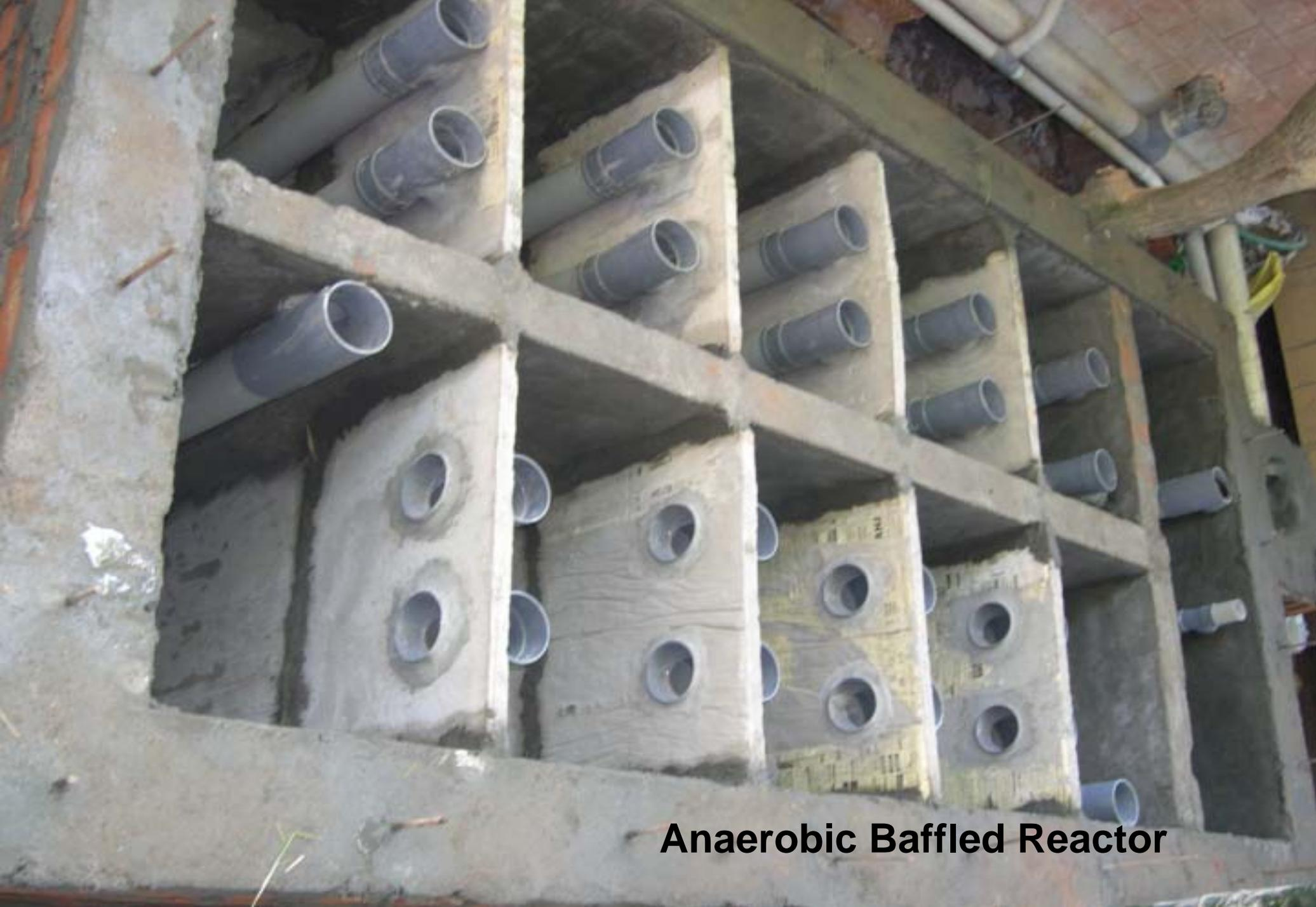
**Anaerobic Baffled Reactor**
